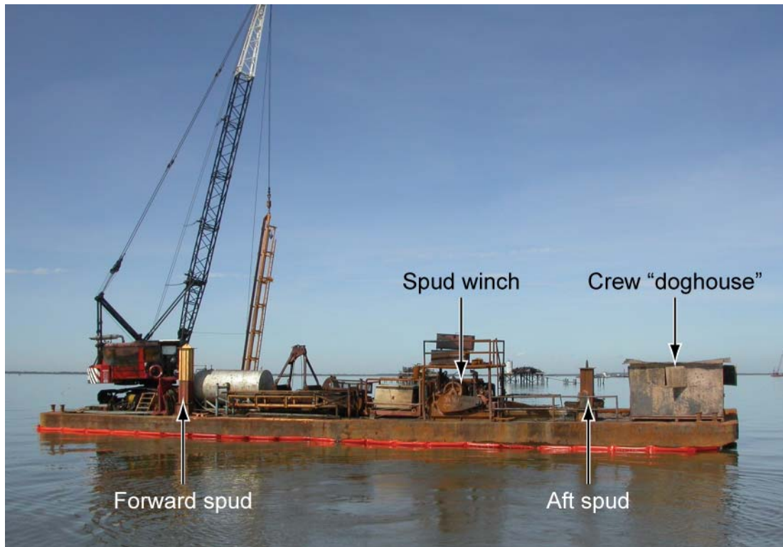
Figure 2. Athena 106 after the fire. The construction barge was equipped with two mooring spuds (shown in the lowered position), both on the port side, one forward and one aft, controlled by a single winch. At the front of the barge was the crane used to hoist and position pilings for driving or to maneuver them to a barge alongside for storage.
