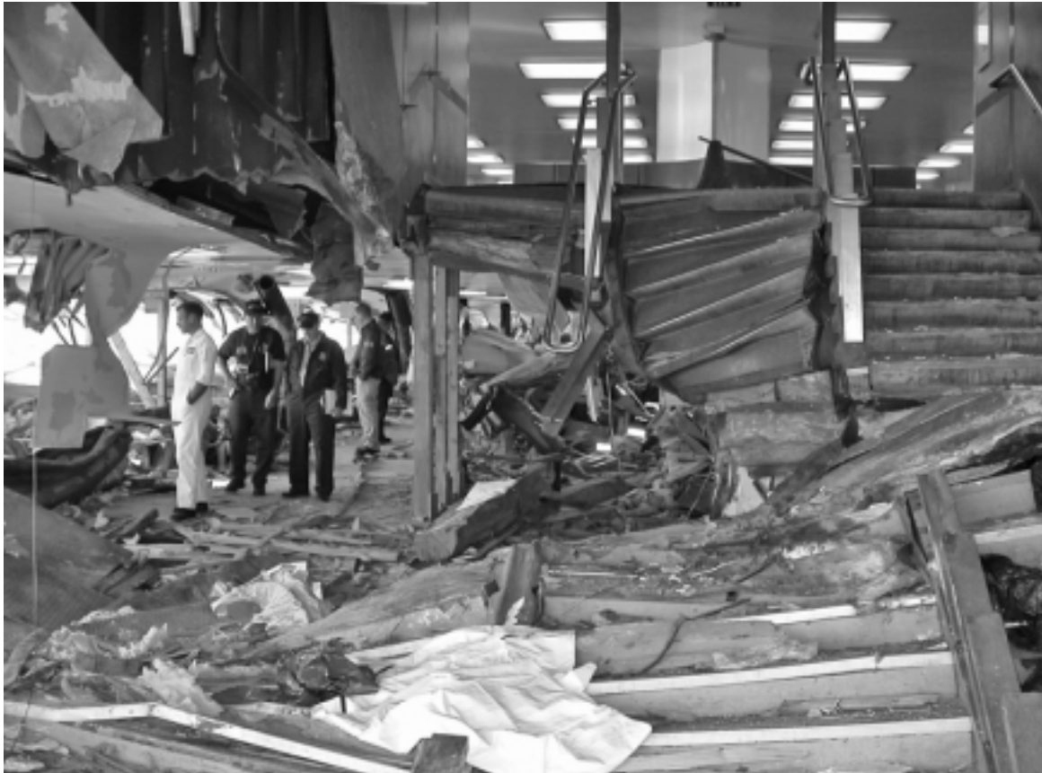
Figure 9. View of damage to New Jersey side of main deck showing collapsed stairway to saloon deck, destroyed columns, crushed seats, ruined ceiling panels, dislodged cables and fixtures, debris, and other destruction.
